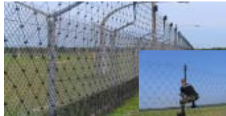
Fiber Optic Security Fence
